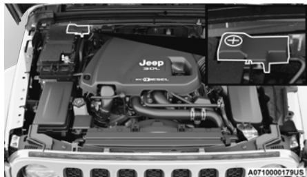
Positive (+) Battery Post – Diesel Engine
